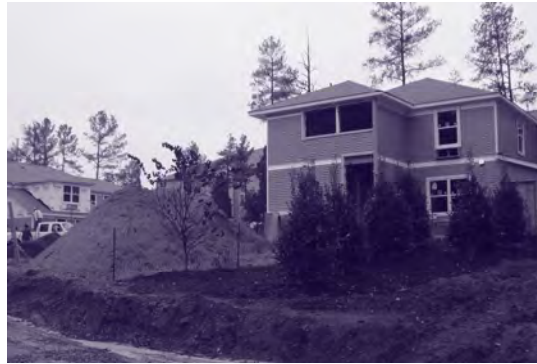
A recent photo of progress at Williams Square.
