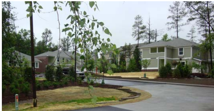
Housing for New Hope’s Williams Square Apartments: twenty-four units of permanent supportive housing and a 2,400 square foot community center, which has a multi-purpose space for tenants and guests, as well as office space for on-site management.
